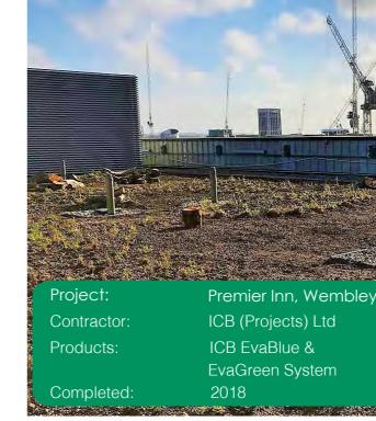
The brief provided to ICB was to create a blue roof which was capable of restricting the flow of rainwater during storm conditions to ensure that the building did not exceed its peak design flow rate of 42I/s to the local sewerage system. In addition to this, a minimum, 350m<sup>2</sup> biodiverse roof area was needed to meet BREEAM.
