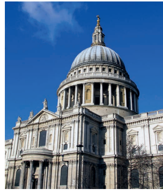
Wall System, St Paul's Cathedral, London
