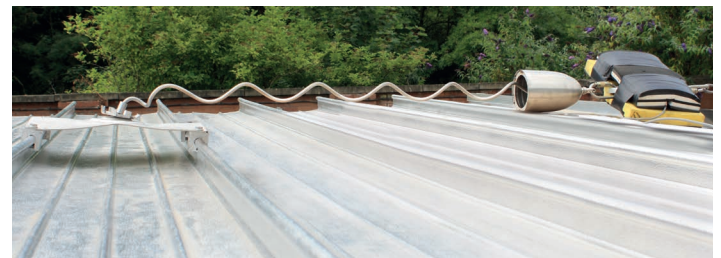
Testing Aluminium Standing Seam
