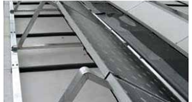
Picture 2: ICB - SOLAFIX as a base for photovoltaic panels
