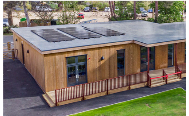
Picture 2: ICB - SOLAFIX as a base for photovoltaic panels
